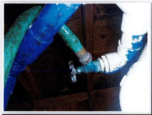
Hose bibb with no vacuum breaker - hose is used to dilute chlorine solution
