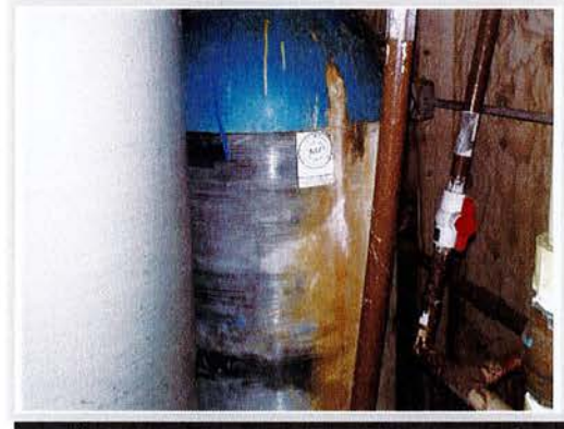
Ion exchange tank
