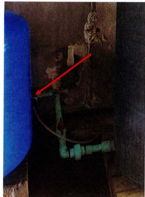
Picture 11. The chlorine injection point is not properly color-coded.
