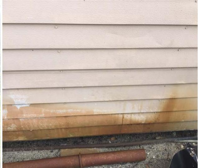
Stain from water sprinklers on gate & rust on shed– needs to be addressed prior to painting
