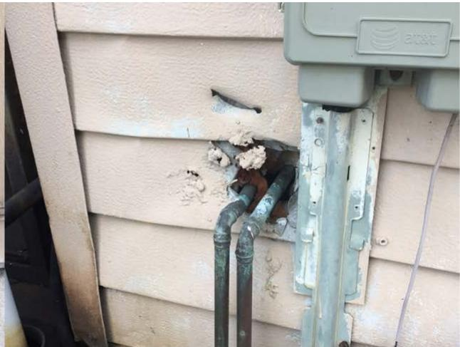
Damaged Metal Siding on Shed – needs to be addressed prior to painting
