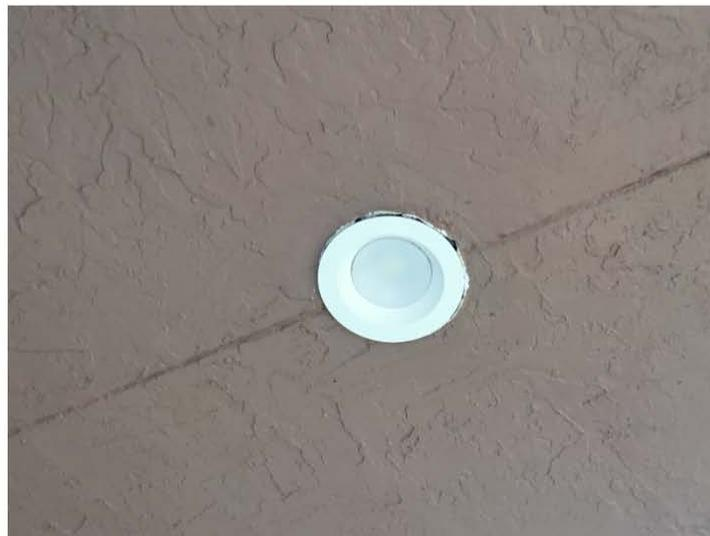
Opening around mounted light on exterior ceiling – needs to be addressed prior to painting
