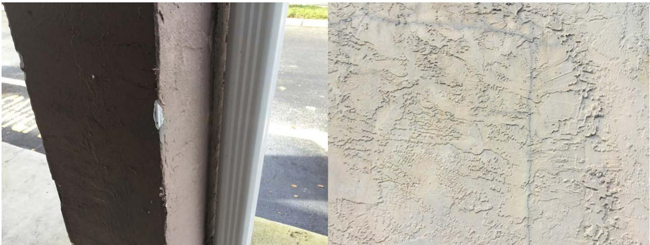
Damaged Stucco, exposing cables & large cracks – needs to be addressed prior to painting
