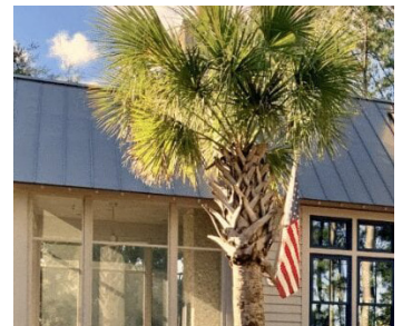
Figure 4.i.4: Example of Florida Vernacular Style "mansard" roof.
