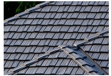
Figure 4.i.1: Example of metal shake roof.
