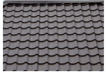
Figure 4.i.2: Example of 5-Tab shingle roof.
