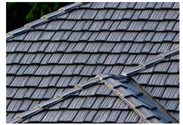
Figure 4.i.1: Example of metal shake roof.
