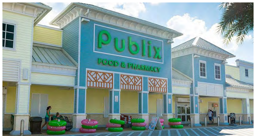
Figure 3.ii.2: There should be no facade that has more than 100' of run without a minimum 16" break in directional or material change.
