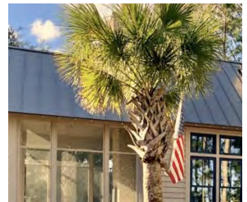
Figure 4.i.4: Example of Florida Vernacular Style “mansard” roof.
