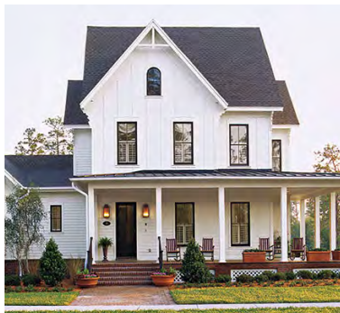
Figure 1.2.iii.2: Example of Florida Cracker Style Architecture.
