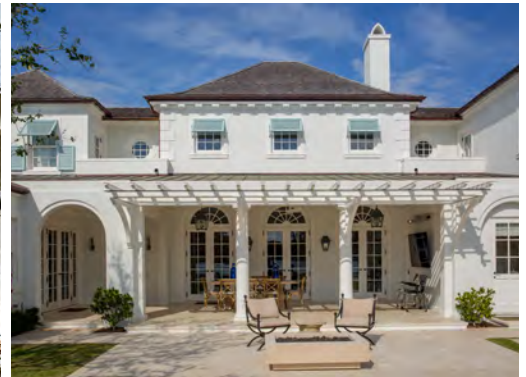
Figure 1.2.ii.1: Example of Caribbean Style Architecture.
