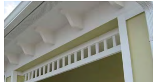
Figure 5.1: Gingerbread trim and/or porch railings, columns or posts must be constructed of wood, aluminum or rustproof metals, composite materials, or other traditionally accepted Florida Vernacular materials to create the appearance of light framed wood construction
