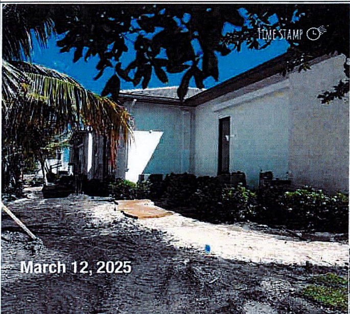
Photo Three Caption: LEFT WEST SIDE
