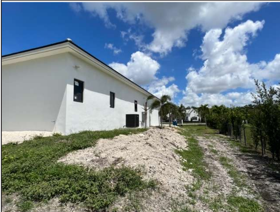
Photo Two Caption LEFT VIEW (04/05/2023)
