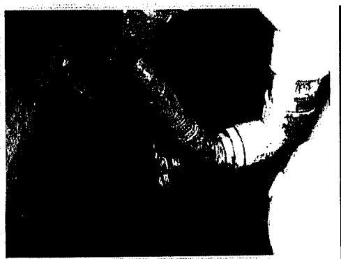
Hose bibb with no vacuum breaker - hose is used to dilute chlorine solution
