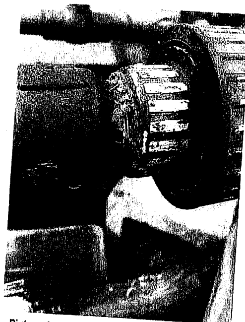
Picture 4. A water leak was observed on downstream of the raw sample tap on the main pump, upstream from the pressure gauge.
