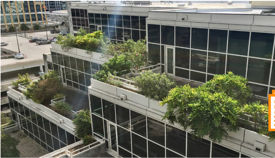
Main Library Exterior Refurbishment
