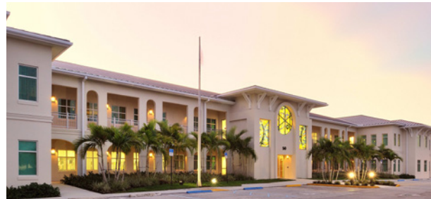
Palm Beach County Four Points Hurricane Hardening, West Palm Beach
