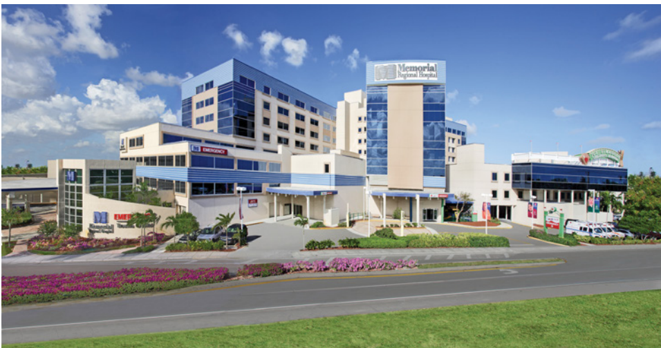
Memorial Regional Hospital Hurricane Hardening
