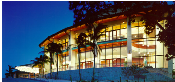
Broward Center for the Performing Arts Hurricane Retrofit, Fort Lauderdale
